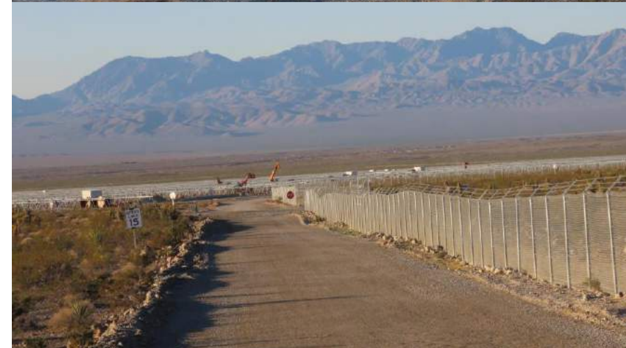
Yellow Pine Solar + Storage
