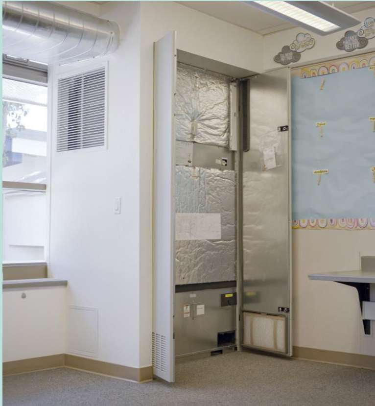
Sunnyvale School District used its $500K grant to install HPWHs
