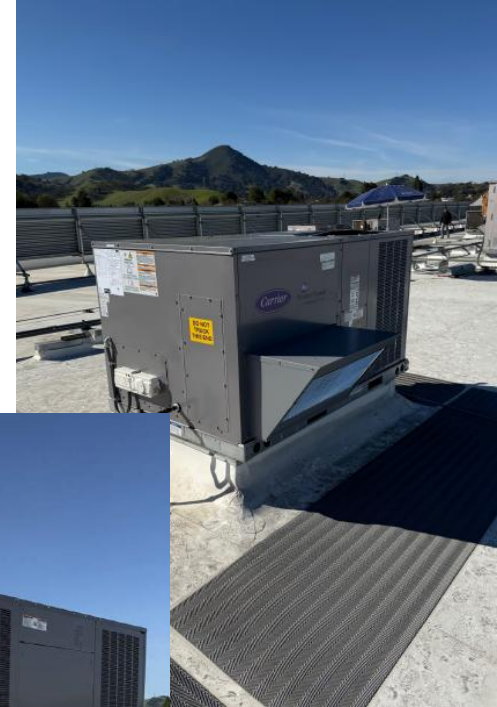
Rooftop Heat Pump HVAC units at Morgan Hill PD
