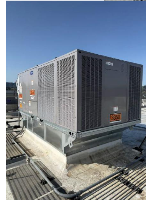
Rooftop Heat Pump HVAC units at Morgan Hill PD
