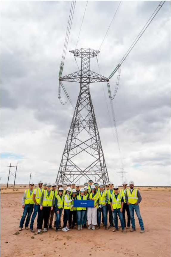
SunZia Wind & Transmission
